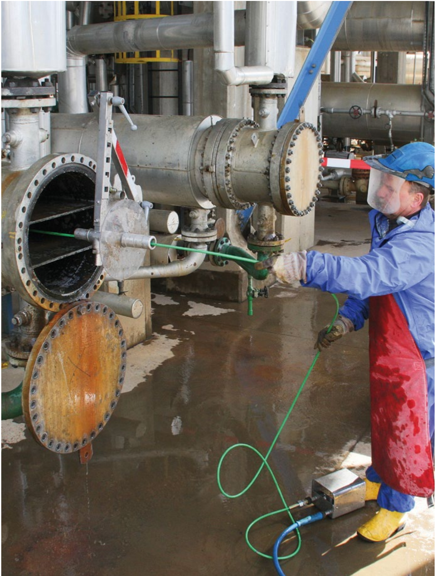
Cleaning heat exchangers
