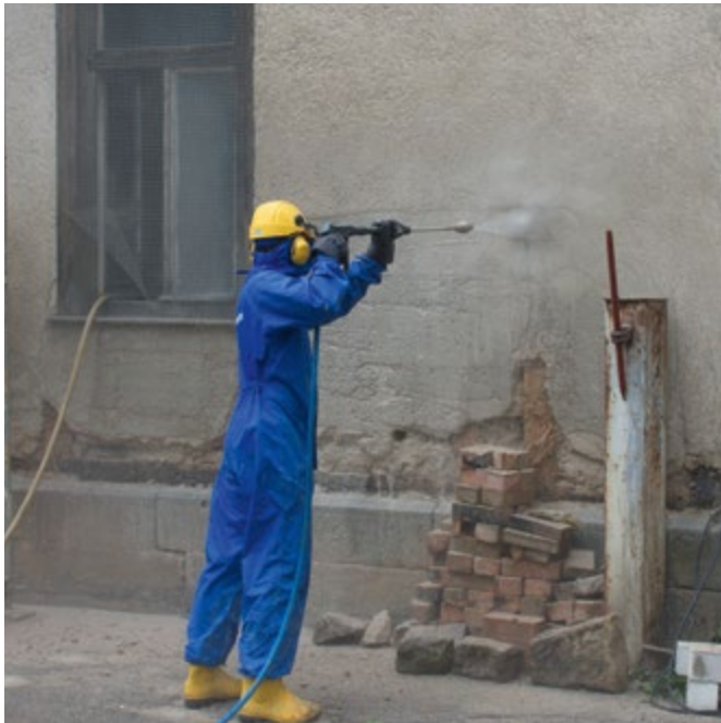
Renovating a facade
