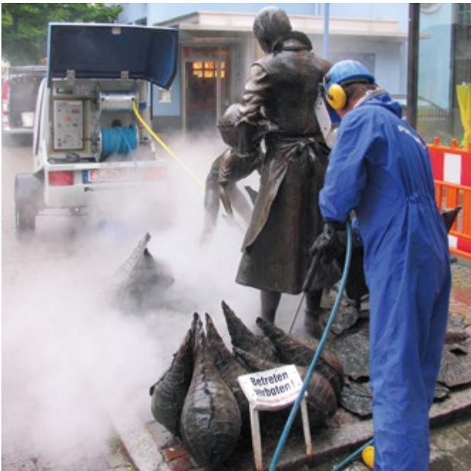
Cleaning a monument
