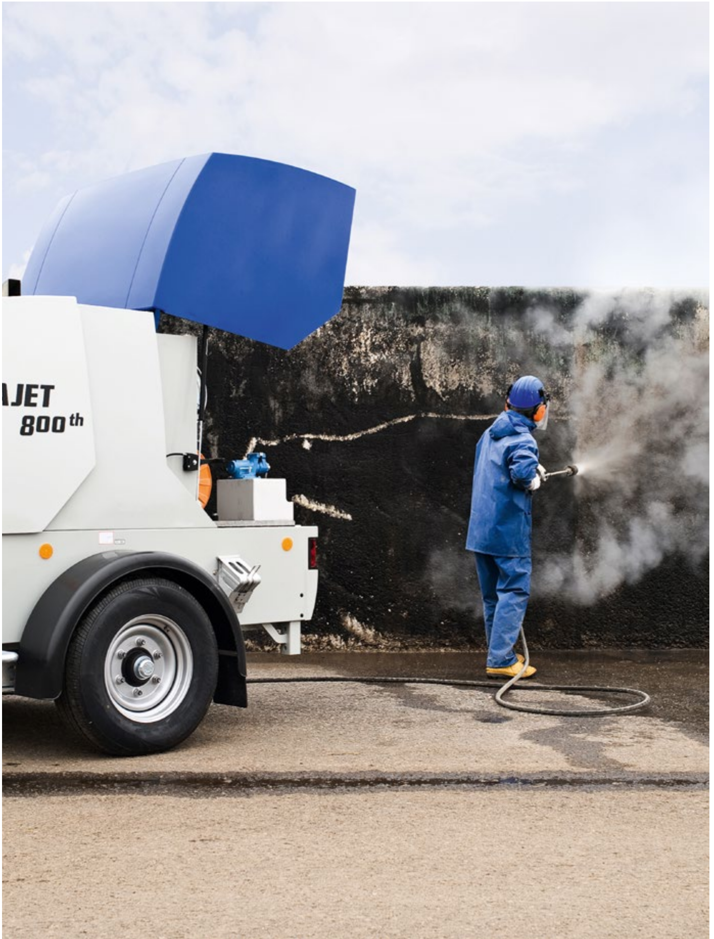
Restoring a bunker silo
