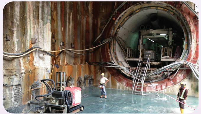
Hydrodemolition technology can reduce labour costs in tunnelling projects by eliminating the need for jackhammer operatives.
