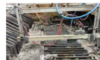
COKE AND REFRACTORY REMOVAL
