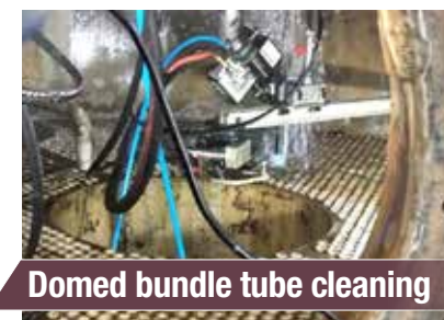
Condenser tube cleaning
