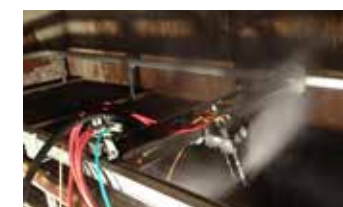
CONDENSER TUBE CLEANING
