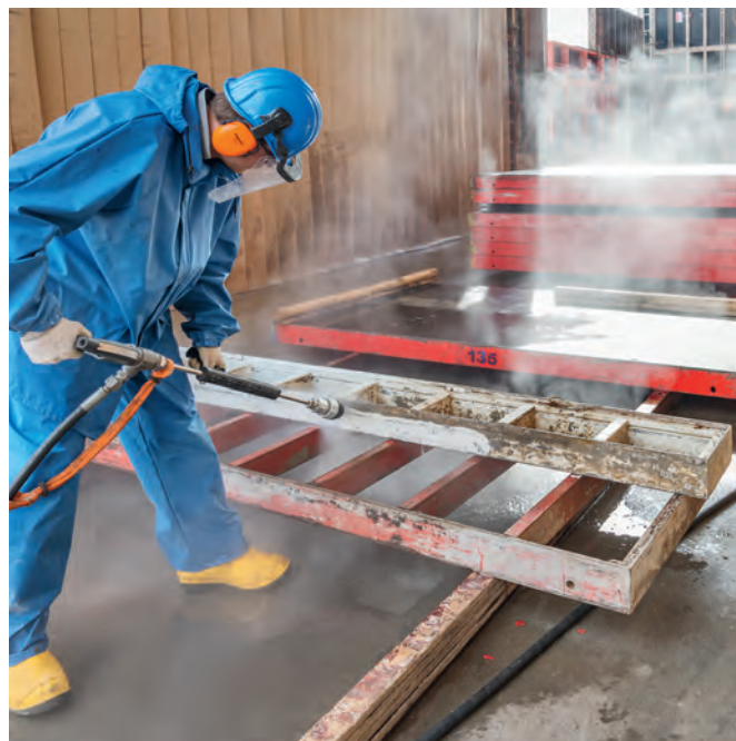
Cleaning shuttering
