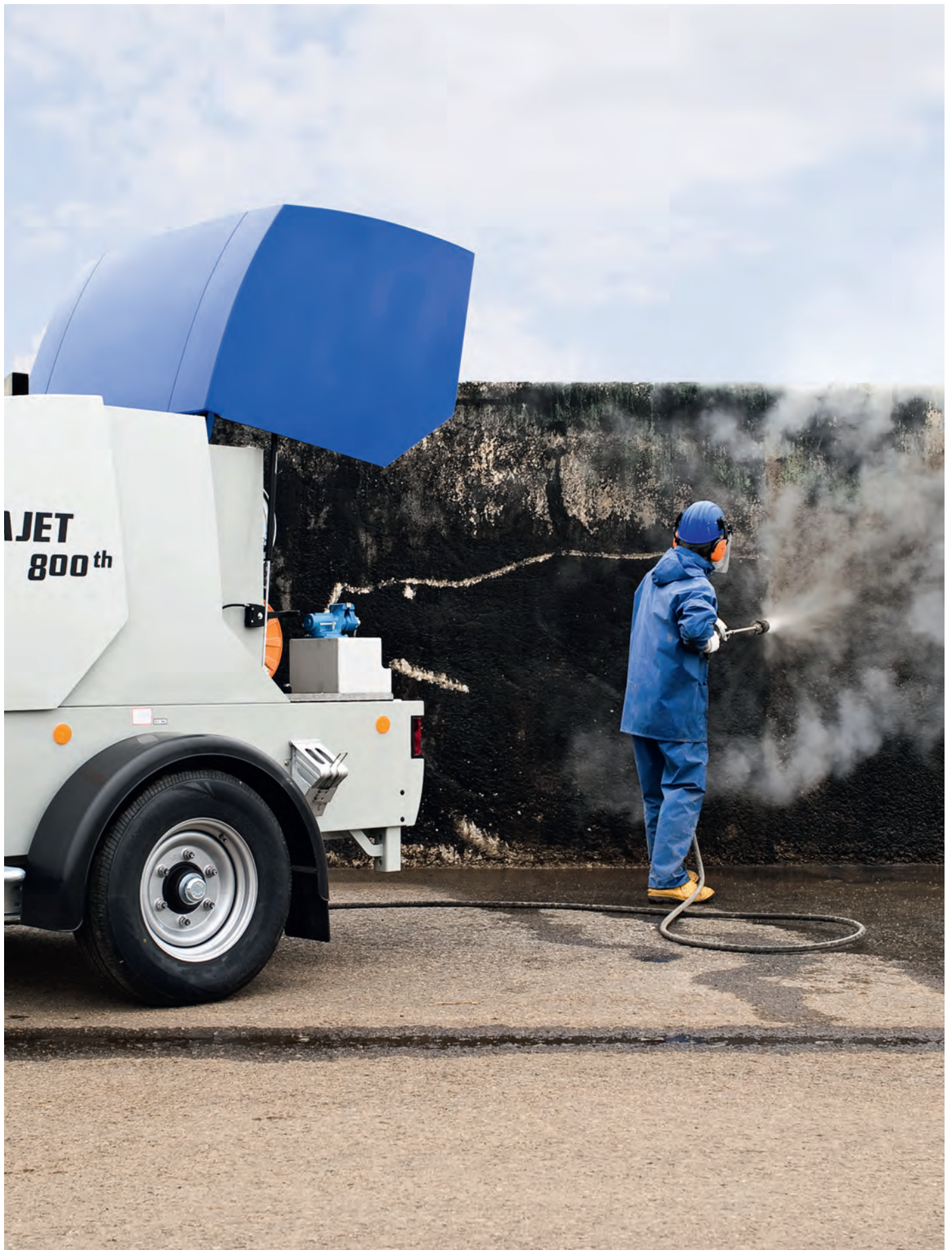
Restoring a bunker silo
