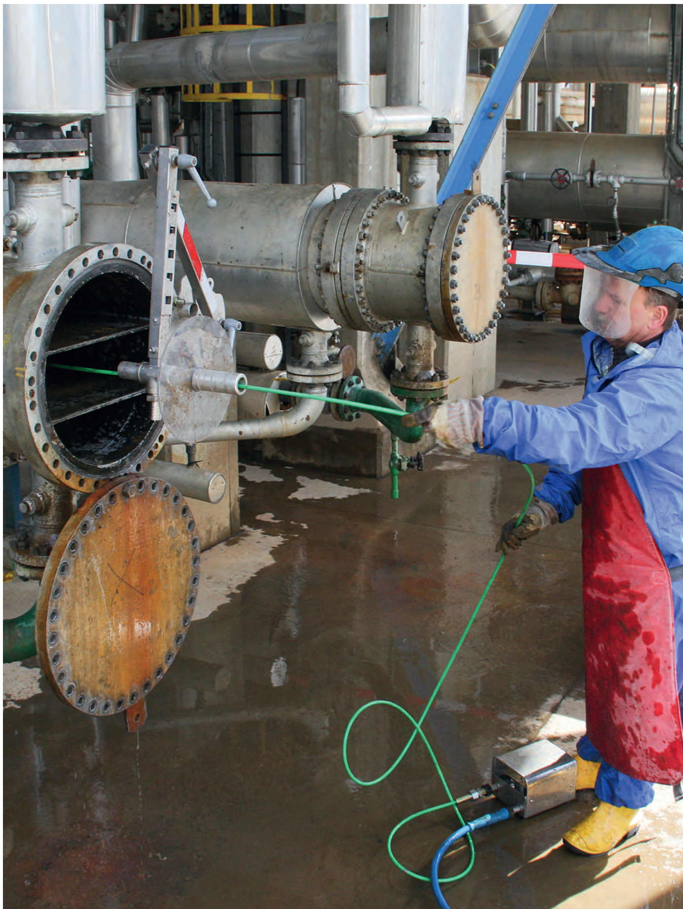
Cleaning heat exchangers
