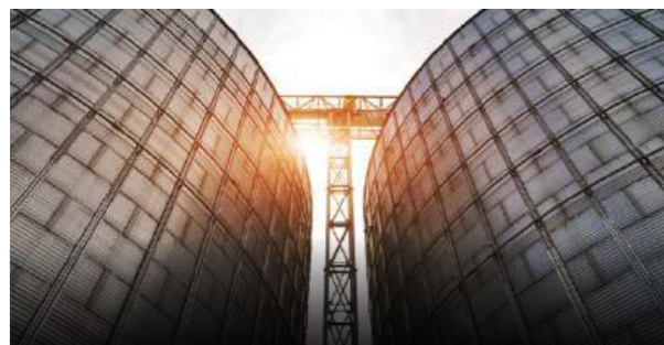
Tank & Vessel Cleaning
