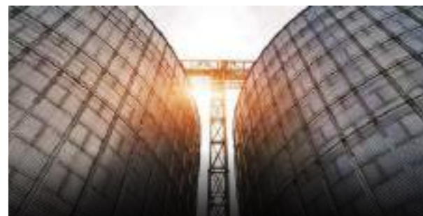
Tank & Vessel Cleaning
