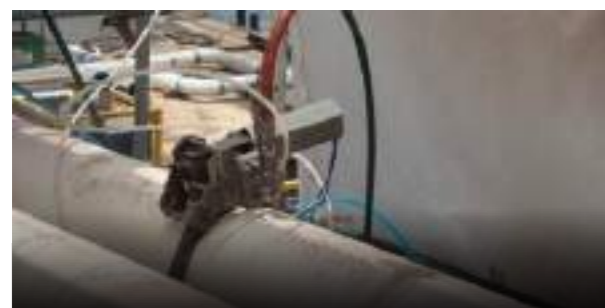
Abrasive Cold Cutting
