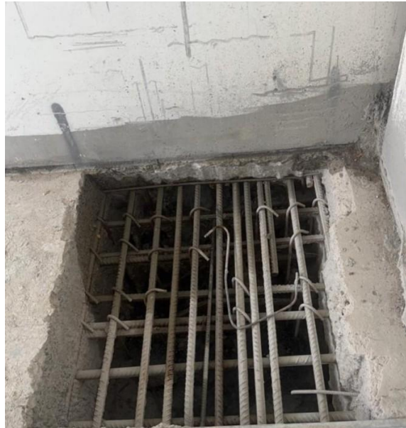
Figure 3 — Completed trench section with clean rebar exposure and defined concrete edges
