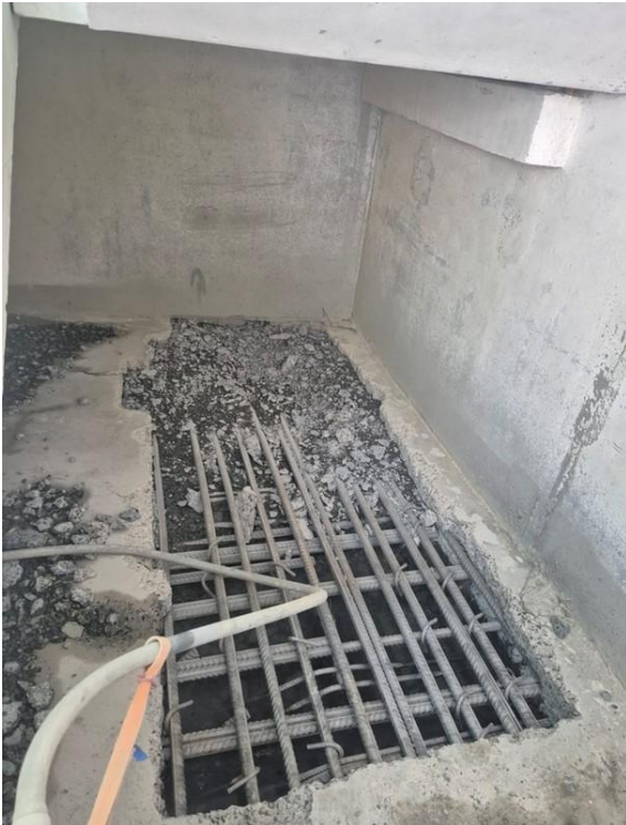
Figure 2 — Exposed rebar during cutting, demonstrating zero damage to reinforcing steel
